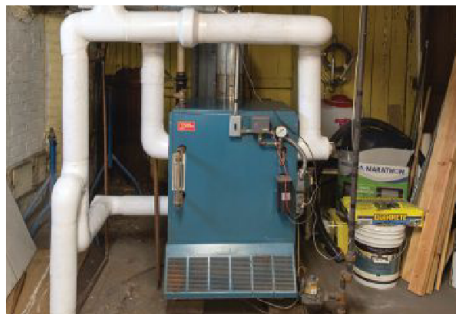
The boiler's new pipe wrapping provides a more comfortable work area.
