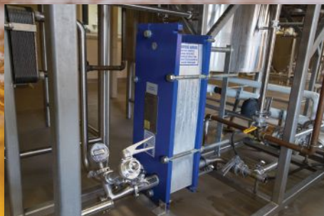
Left to right above: A glycol cooling system chills the beer tanks and the draught beer cooler. Brewery Vivant's delicious menu items are prepared by Adam Lance on a natural gas stove for optimal energy efficiency. The heat exchanger reduces energy needs by transferring energy from one area to another.
